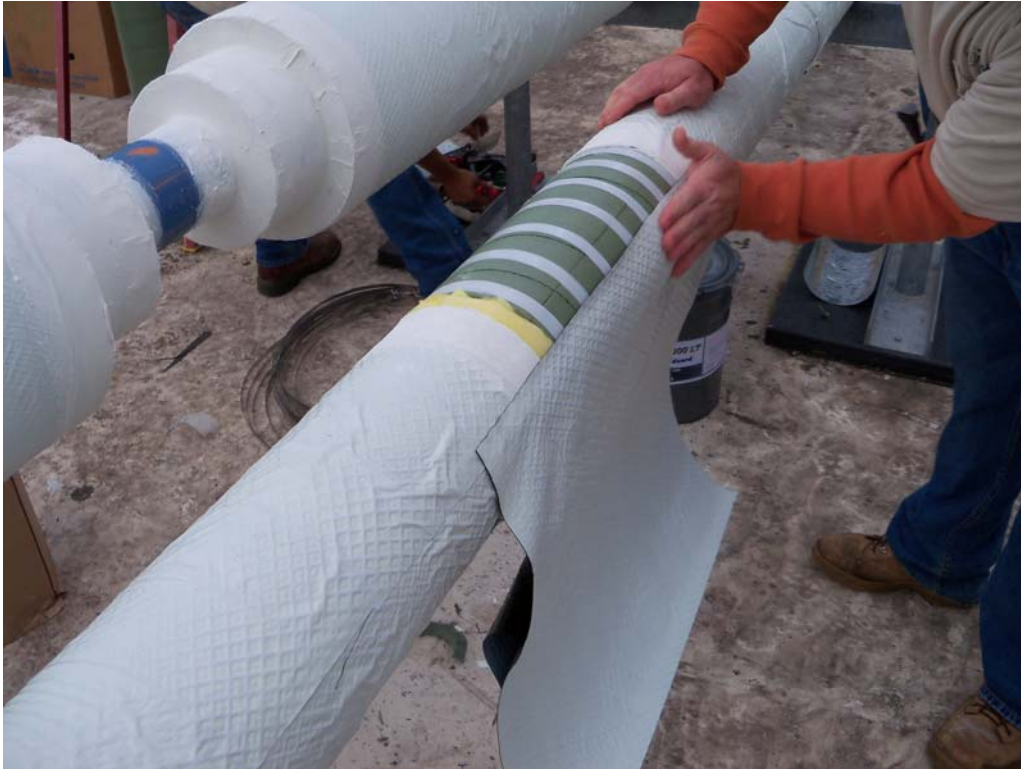
Double layer expansion joint assembly, vapor retarder being installed.
