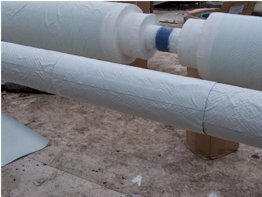
Double layer expansion joint assembly completed, location to be identified on jacket.
