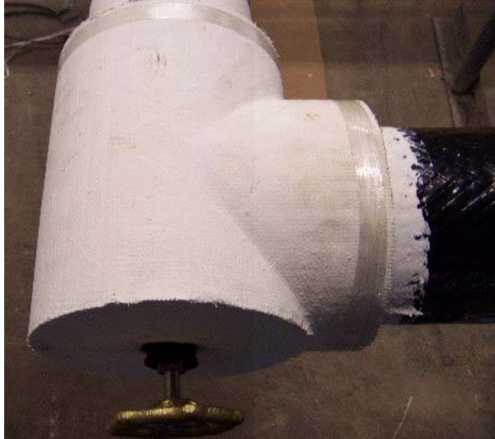
Angle valve installations (secure and tape).
