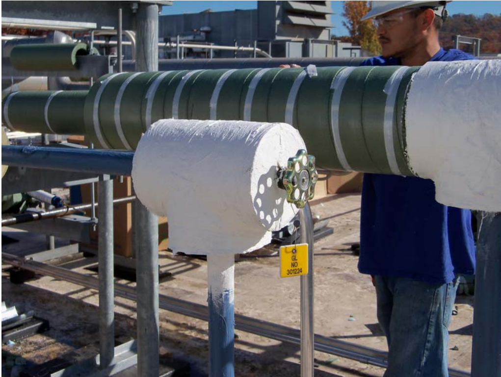
Vapor retarder mastic application completed.
