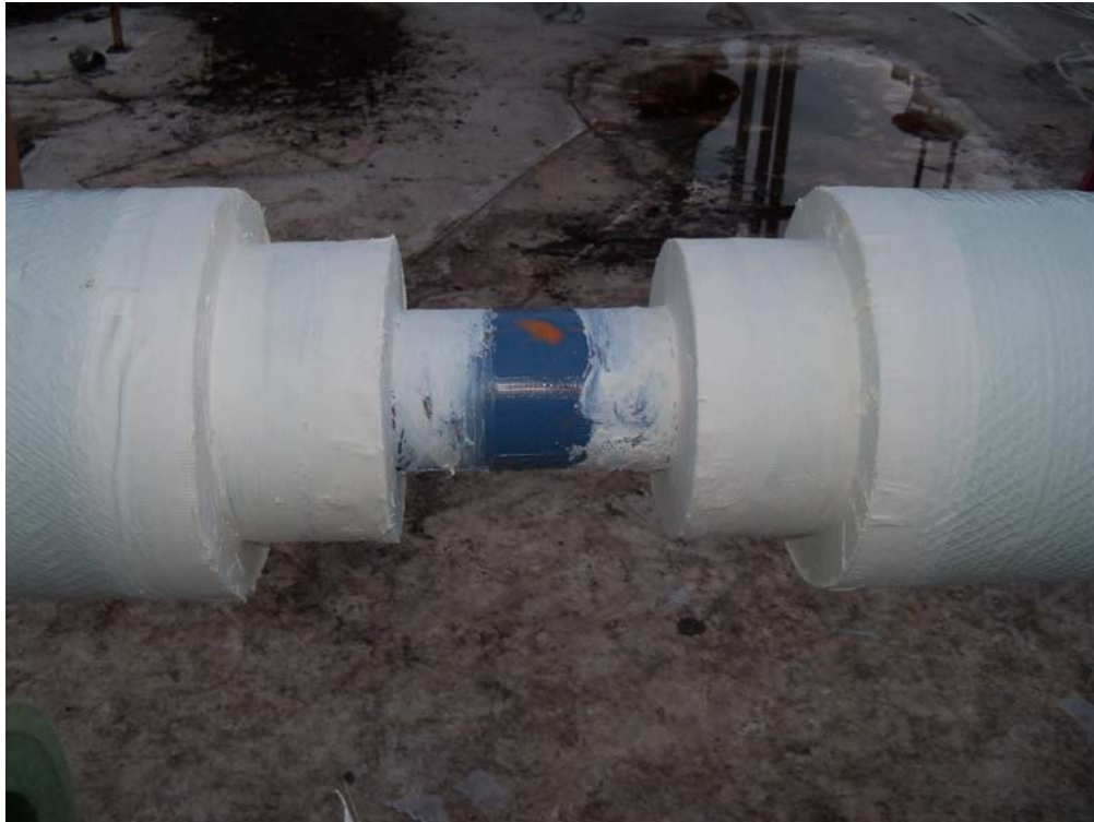
Double layer expansion joint assembly, vapor barrier and mastic / mesh applied.
