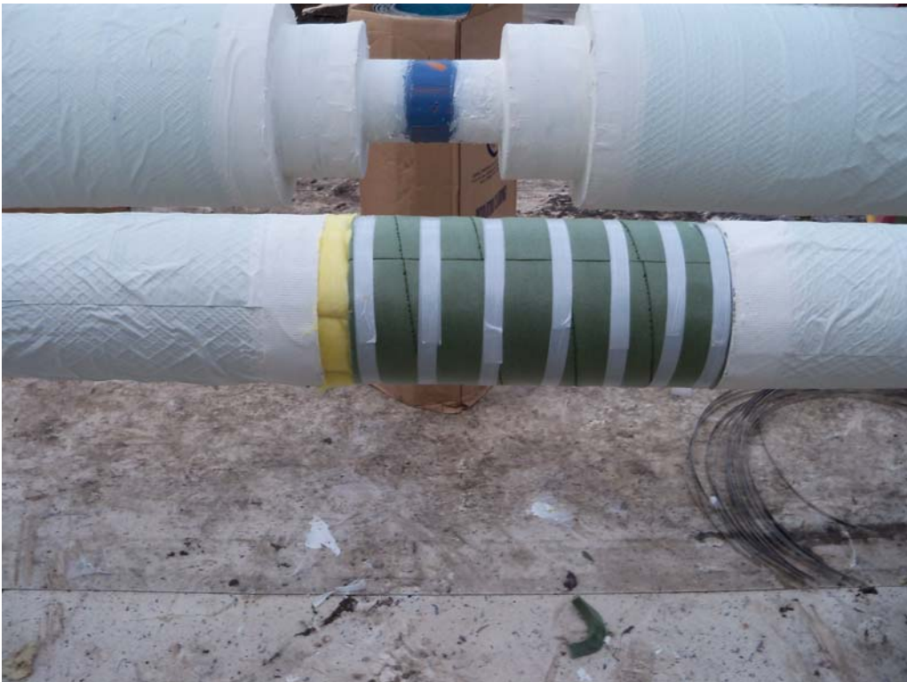
Double layer expansion joint assembly, 15" Cryoflex and 1" fiberglass installed on 2 nd layer.
