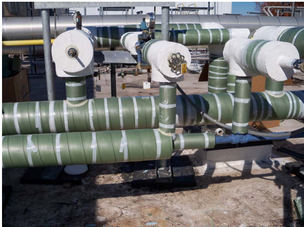
Cryoflex installed on pipes coated with anti-corrosive gel.
