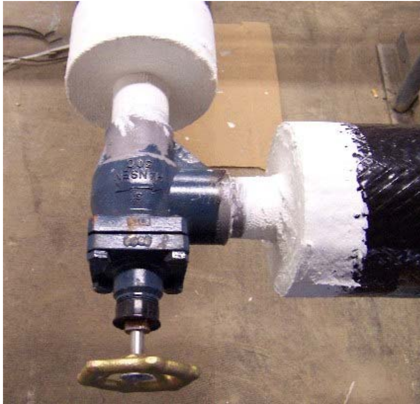
Angle valve installation (vapor barrier applied).
