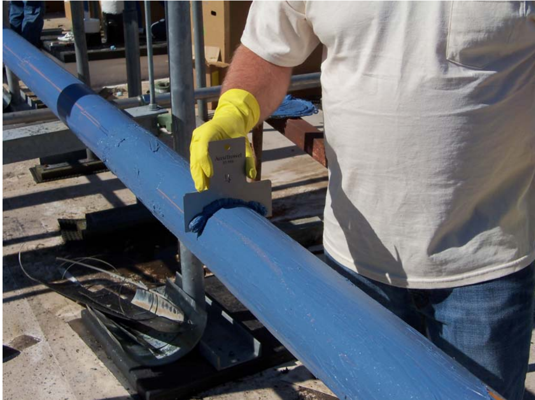
Anti-corrosion gel applied to pipe using an Accutrowel™ screed.
