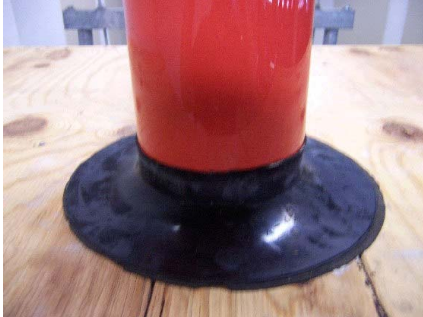
Roof penetration before aluminum cladding.
