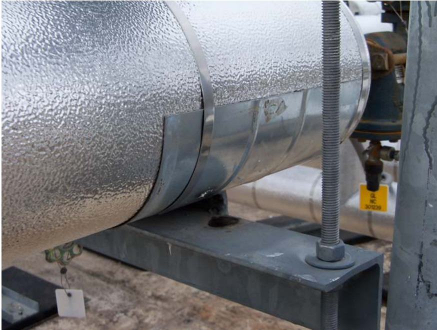
Galvanized saddle banded in place.
