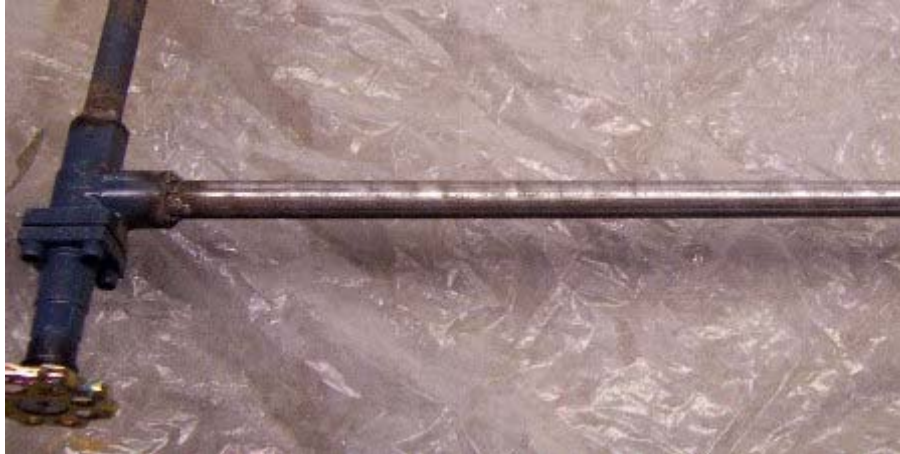
Remove dirt, rust, and scale on all pipes to be primed and painted.
