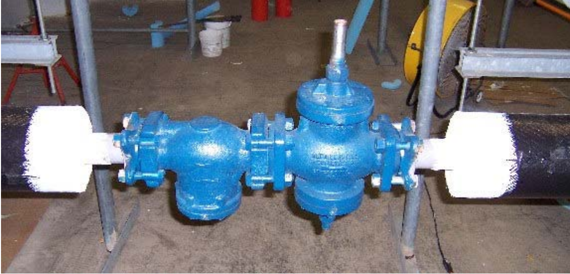
Vapor barrier at control valve.
