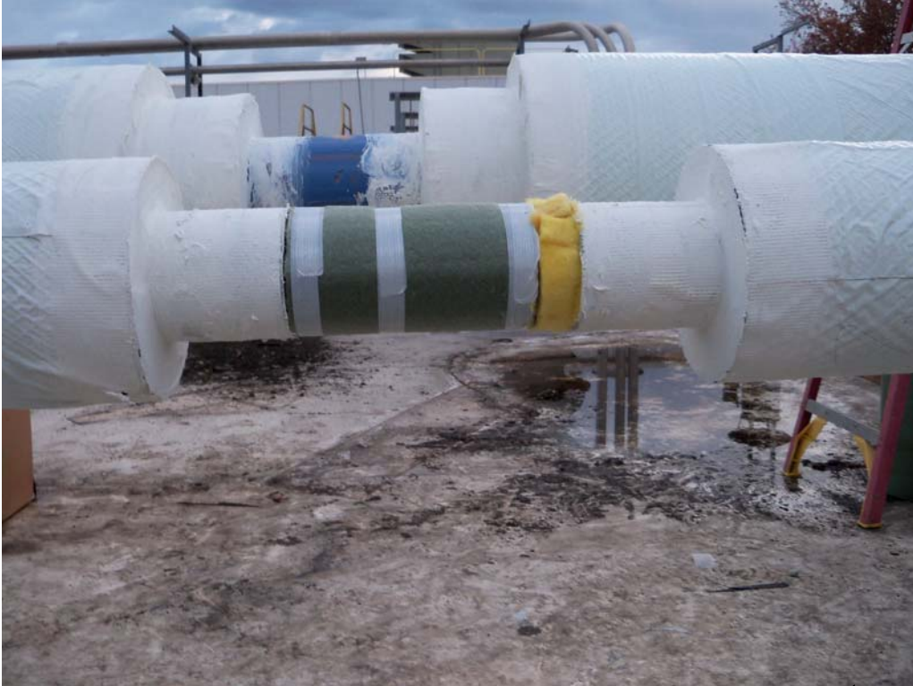
Double layer expansion joint assembly, 7" Cryoflex and 1" fiberglass installed on 1 st layer.
