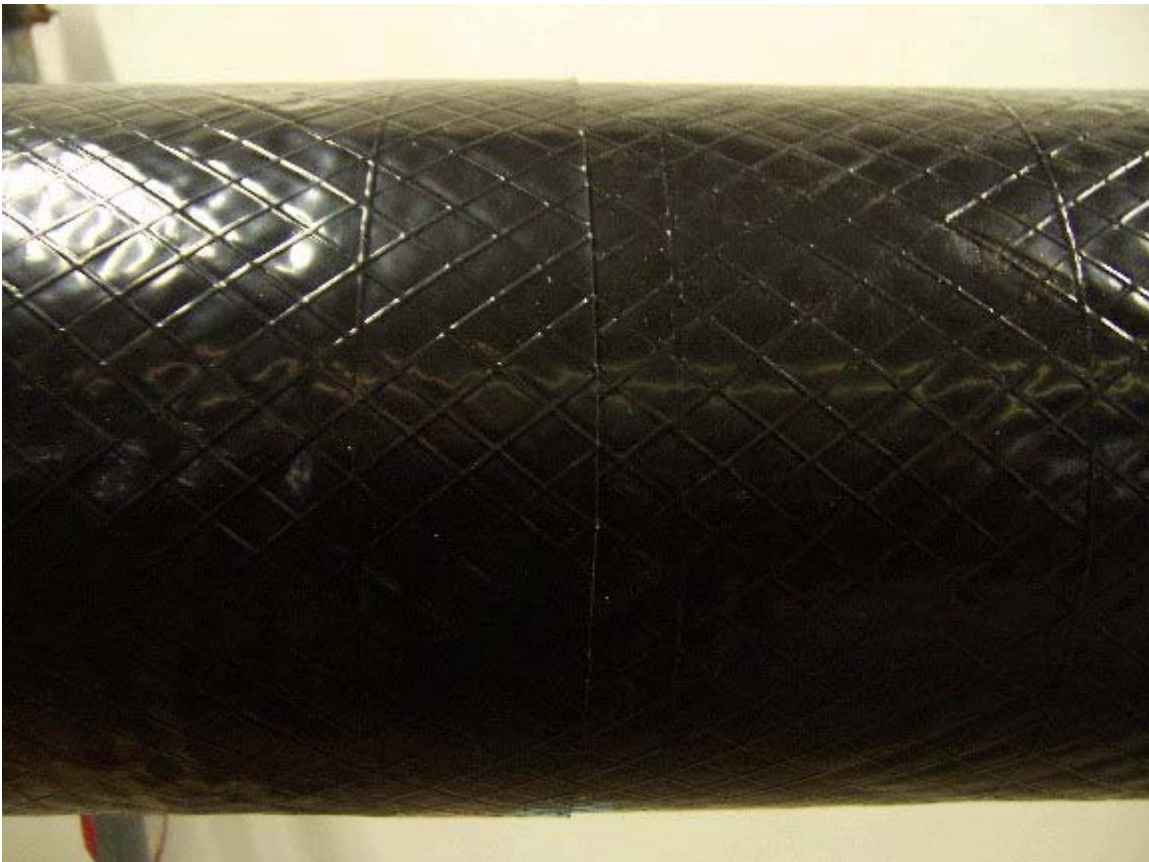
Vapor barrier to be continuous on all insulated piping (Insulrap 30 vapor retarder shown)
