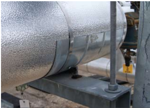
Aluminum (insulation protection saddle, not banded yet).
